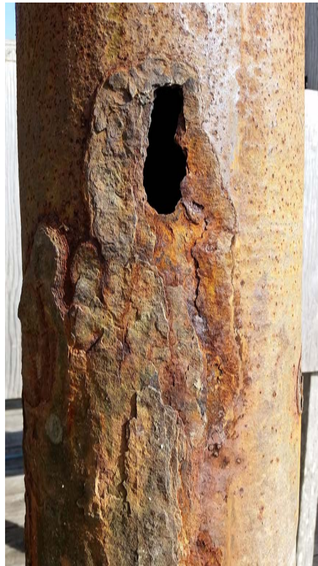
Pile Corrosion
