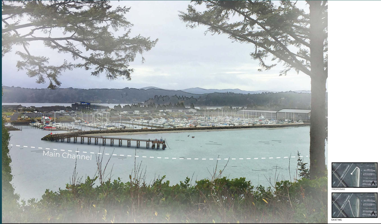
PORT OF NEWPORT PORT OF NEWPORT PUBLIC FISHING PIER | LOOKING SOUTH
