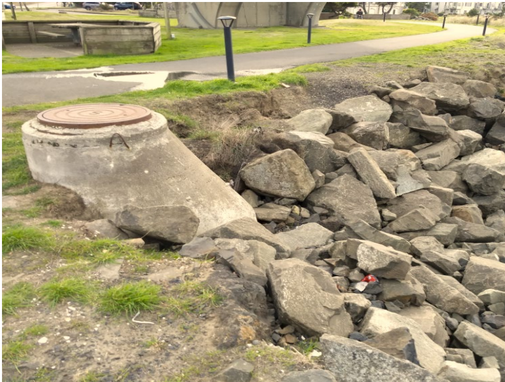
Photo 31 – Manhole and Riprap near Bridge
