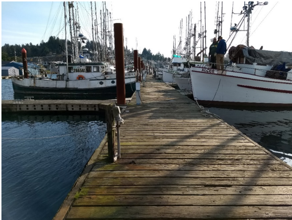
Photo 11 – Port Dock 7 – Wood Floating Dock and Concrete Fingers
