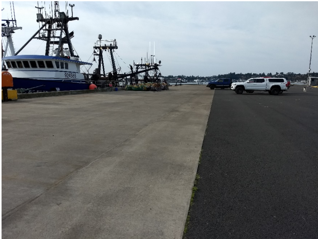
Photo 20 – International Terminal – West Berth
