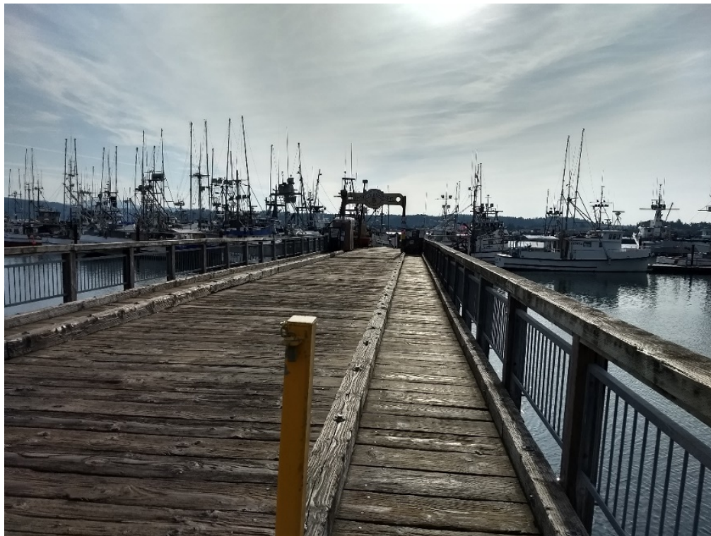
Photo 6 – Port Dock 5, Approach Trestle
