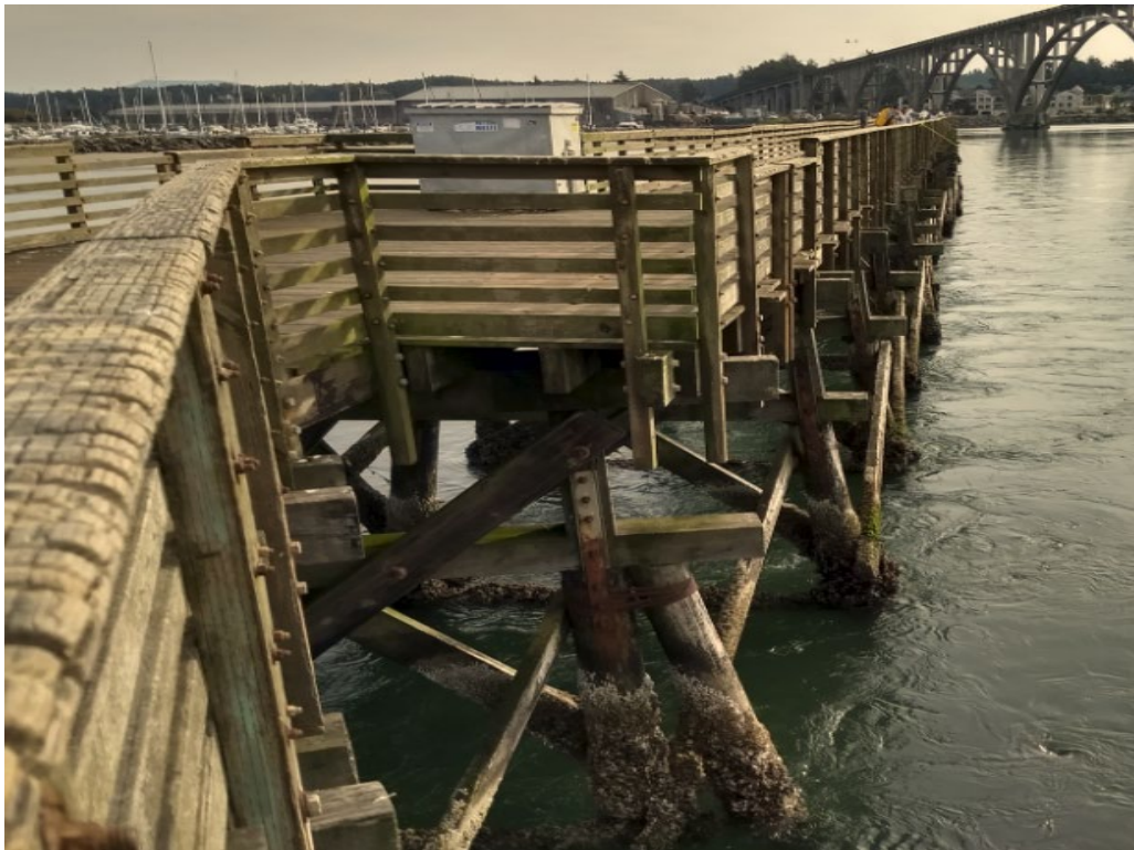
Photo 25 – Fishing Pier – Substructure Support
