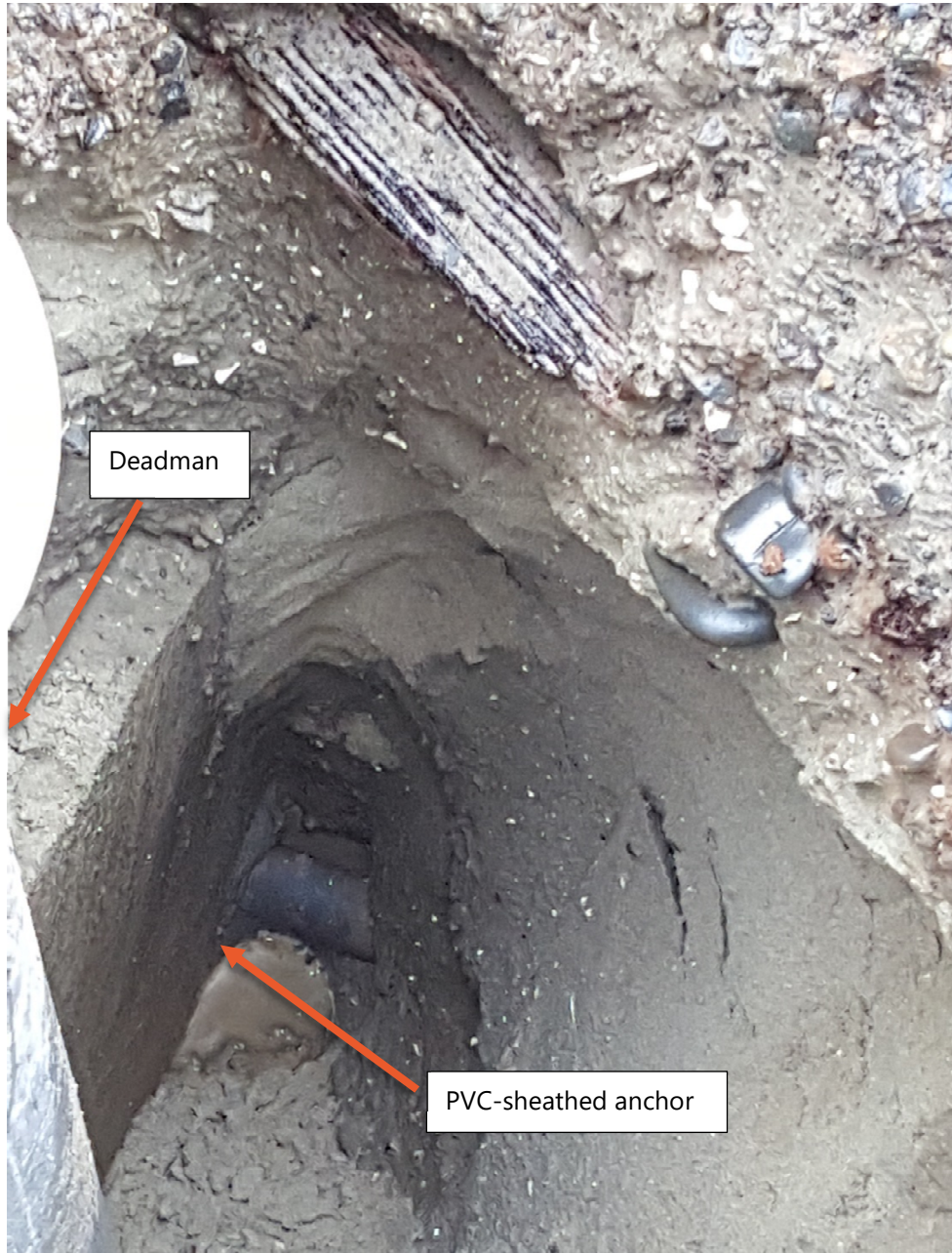
Figure 3. Deadman Tie-back Anchor, Seawall Side
