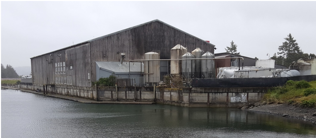
Figure 3-1 Rogue Brewery Seawall
