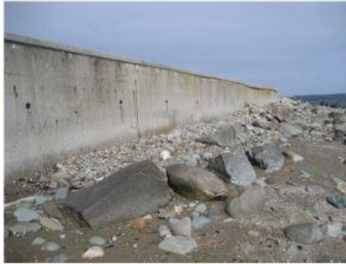
Fig. A-18. Mass concrete seawall
