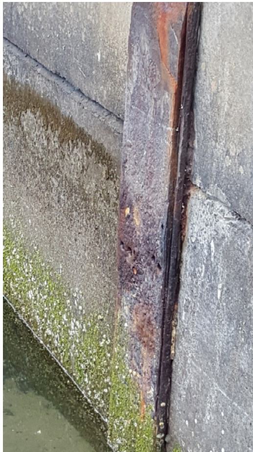
Figure 1. Steel Pile at Splash Zone
