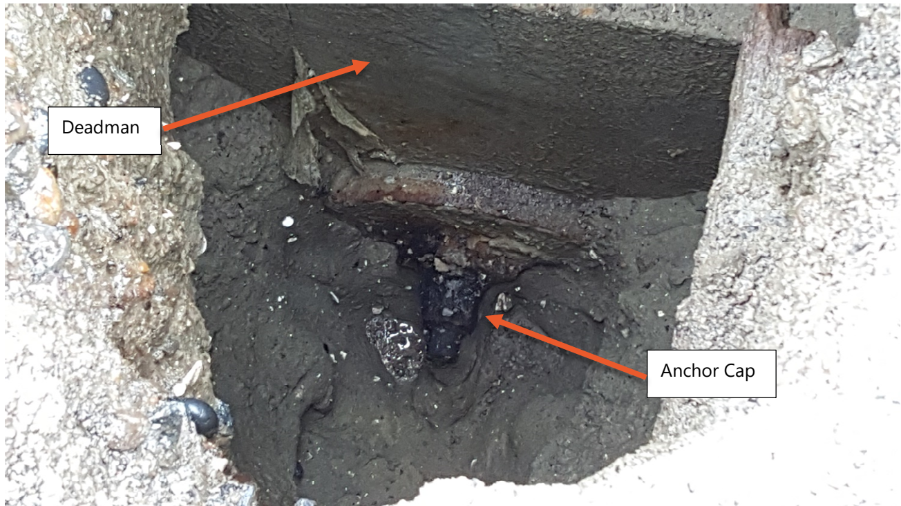
Figure 4. Deadman Tie-back Anchor, Upland Side
