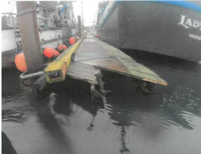
Photo 12: West end of Dock E/F
