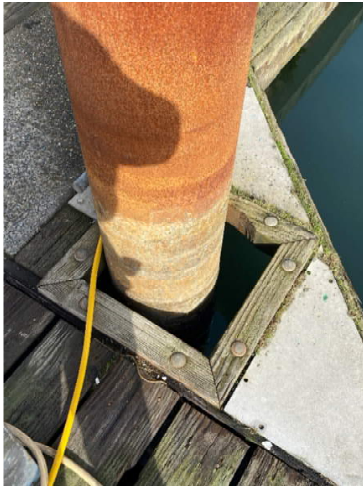
Photo 6: Rub block at piles
