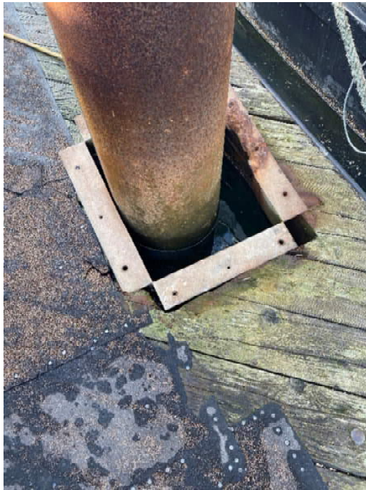
Photo 16: Pile penetration at Dock X between Dock C/D and E/F.
