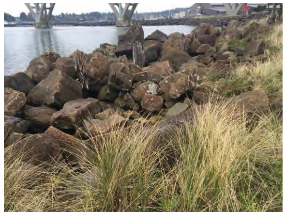
Picture #48. Rock shoring
