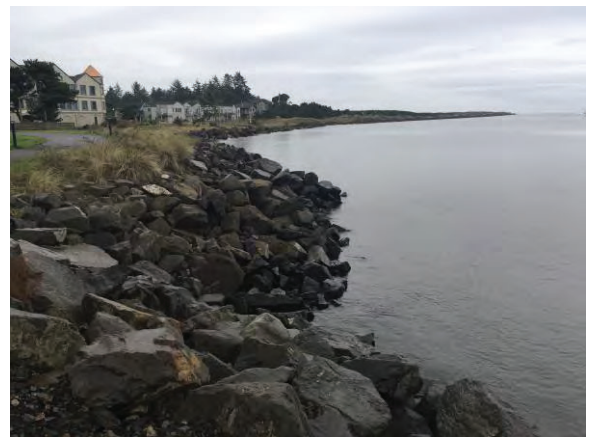
Picture #12. Rock shoring
