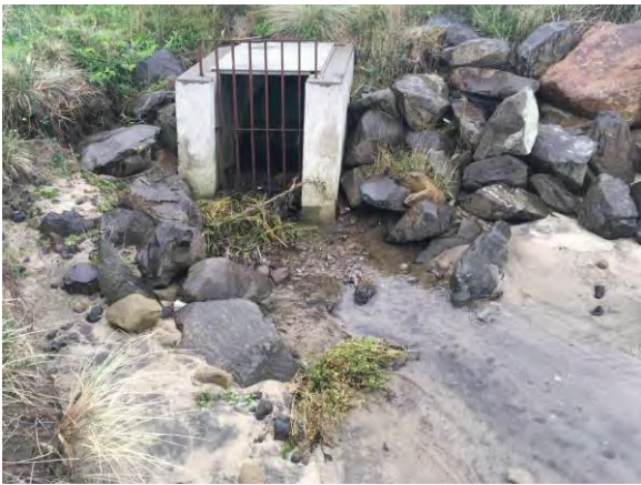
Picture #44. Drain outlet
