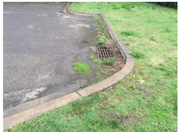
Picture #36. Drain in parking area
