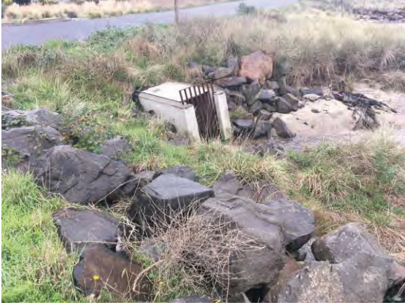
Picture #43. Drain outlet
