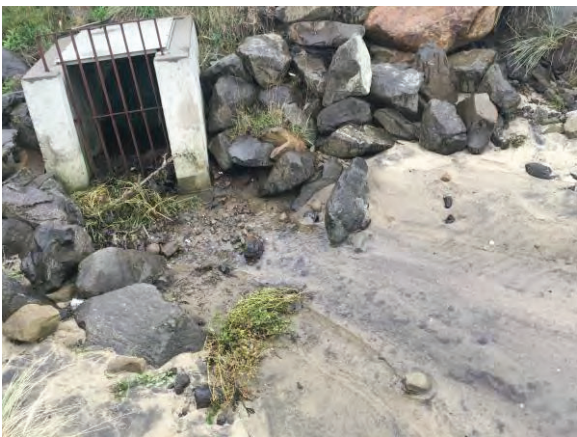
Picture #45. Drain outlet
