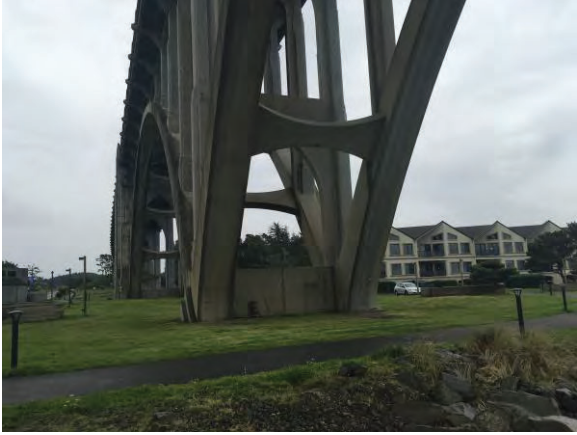
Picture #13. Bridge pier
