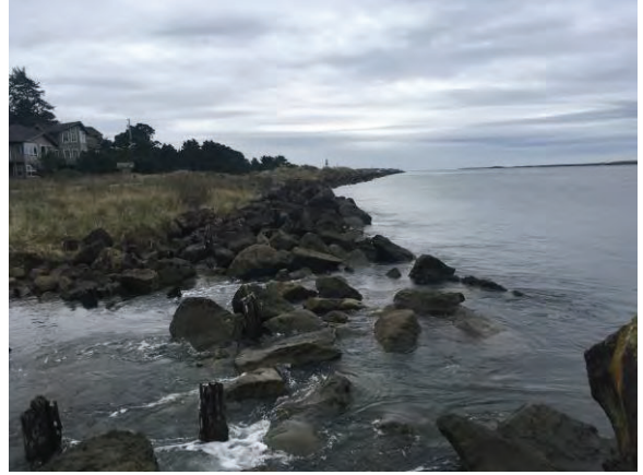
Picture #52. Rock shoring
