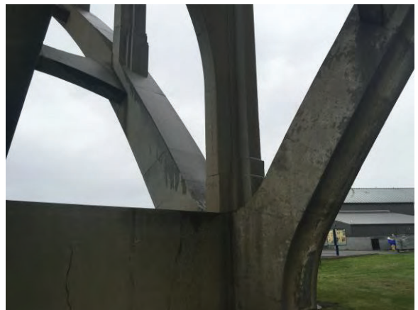
Picture #18. Bridge pier
