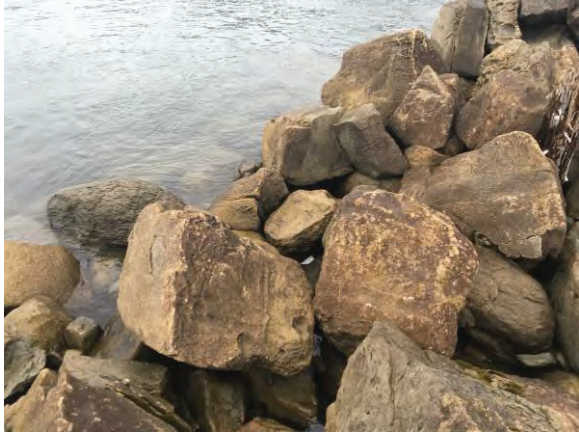
Picture #49. Rock shoring
