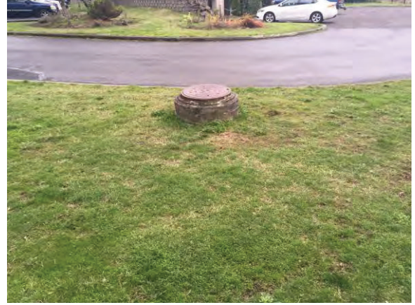
Picture #22. Sanitary sewer manhole
