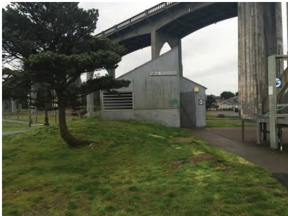
Picture #3. Public restroom near (but outside) the Property
