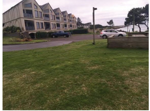
Picture #28. Paved parking area
