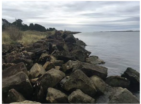
Picture #53. Rock shoring
