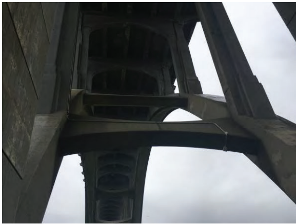
Picture #26. Bridge pier
