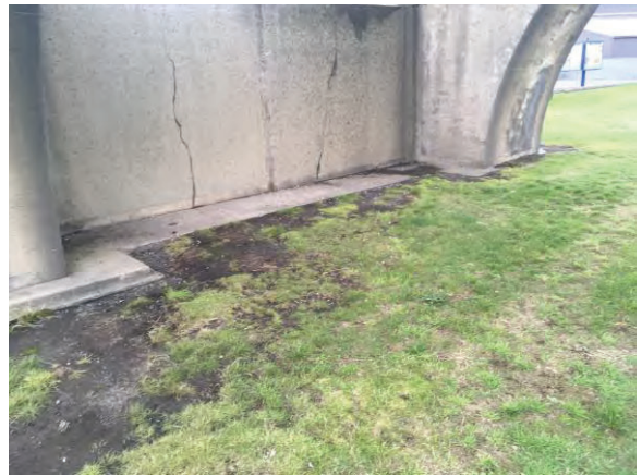
Picture #17. Bridge pier
