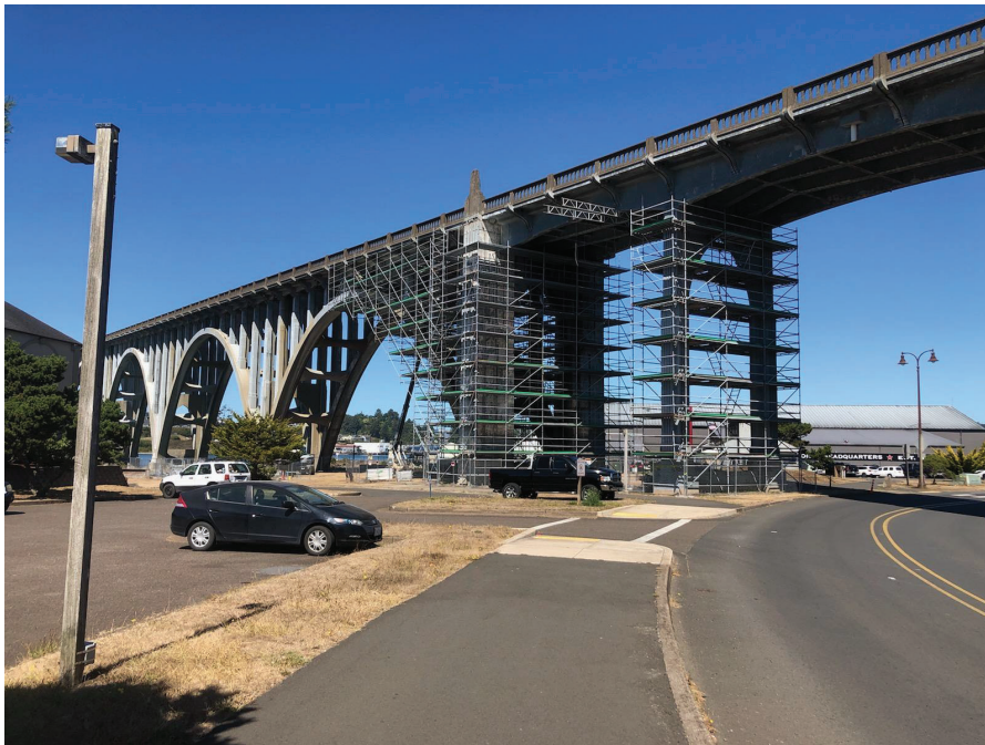
Yaquina Bridge, Newport - ODOT Scaffolding looking northeast
