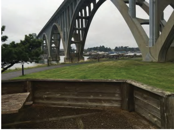
Picture #31. Yaquina Bay bridge
