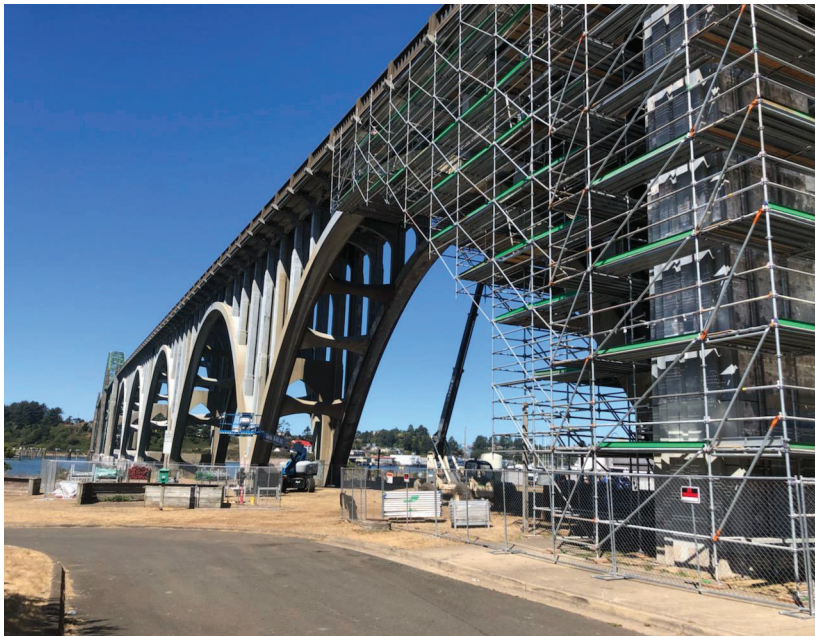
Yaquina Bridge, Newport - ODOT Staging area and scaffolding - looking north
