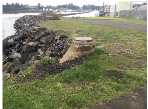
Picture #11. Sanitary sewer manhole
