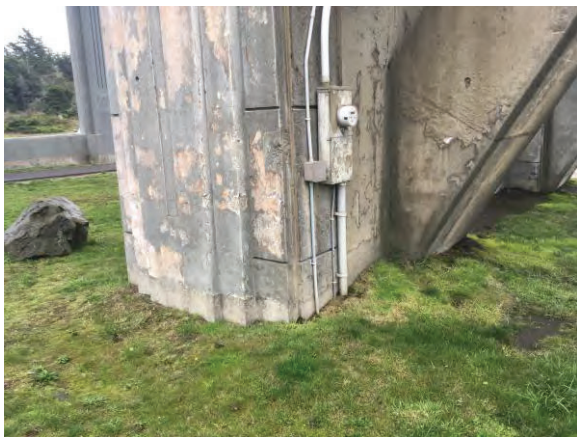
Picture #27. Bridge pier
