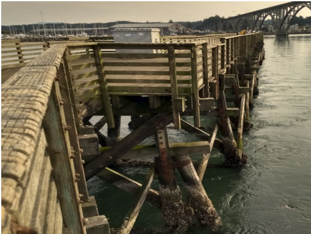
Photo 25 – Fishing Pier – Substructure Support
