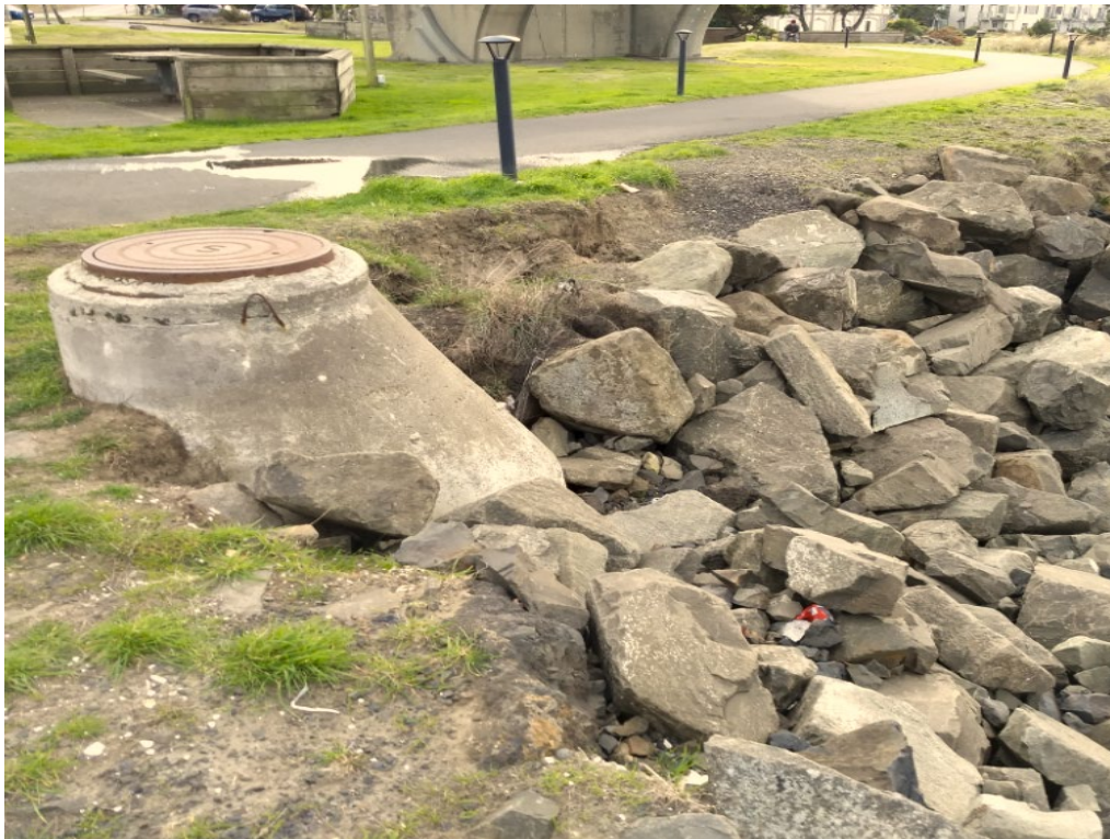
Photo 31 – Manhole and Riprap near Bridge
