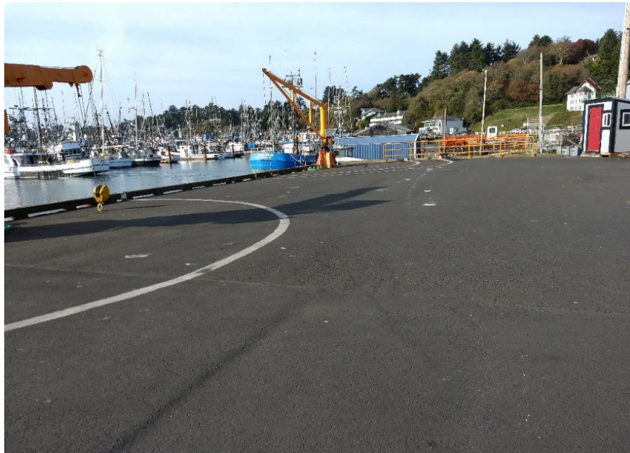
Photo 13 – Hoist Dock – Swing Crane
