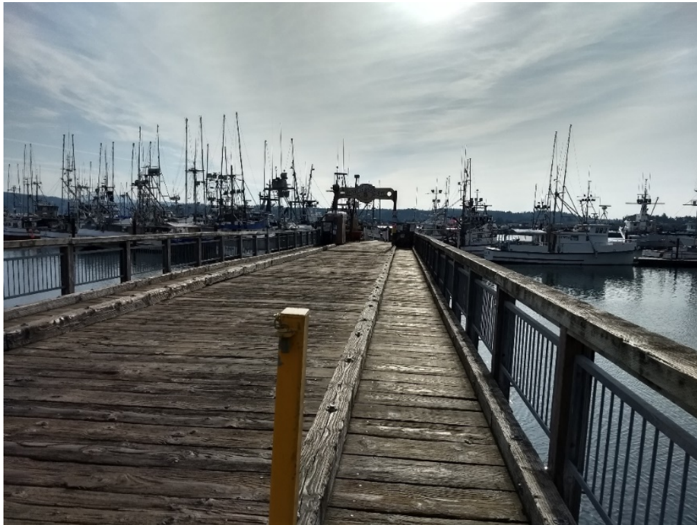
Photo 6 – Port Dock 5, Approach Trestle
