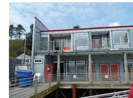
MULTI-STORY BUILDINGS Anchor Pier - Newport, OR
