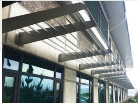
NATURAL DAYLIGHTING NOAA MOC-P Facility - Newport, OR
