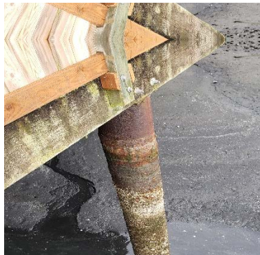
Northern Piling From Gangway
