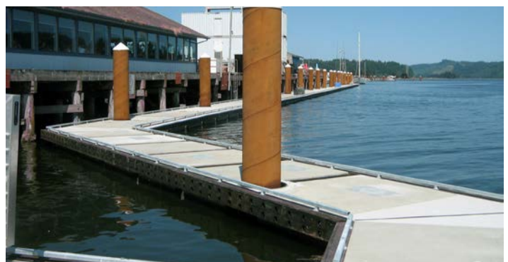
DOWL worked closely with the Port of Siuslaw to develop project goals and conceptual designs for floating dock facilities that equally serve both the commercial fishermen and recreational users.
