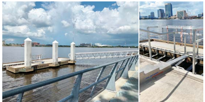
HDR provided design, permitting, and construction services for the Southbank Kayak Launch in Jacksonville, Florida, which optimized user accessibility features.
