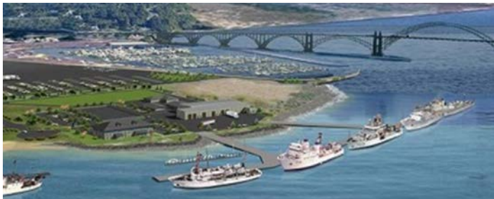
PHS coordinated extensively with USACE on the NOAA MOC-P project.
